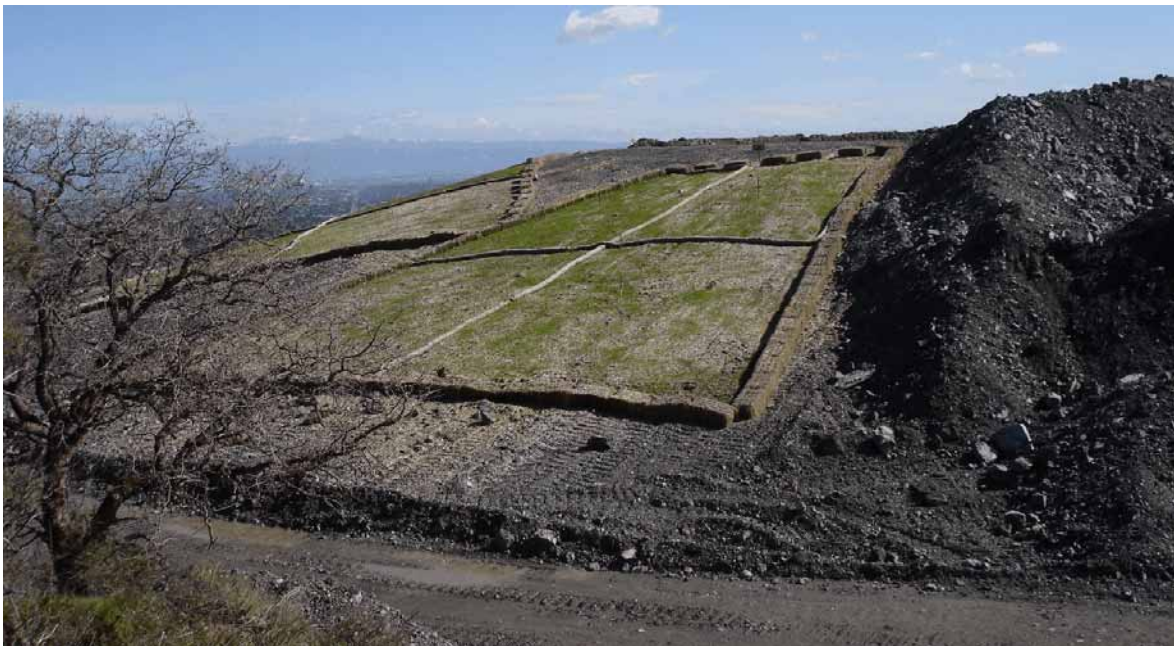
Top: Test plot construction at Yeager Yard: Blending soil materials (October 17, 2008)
