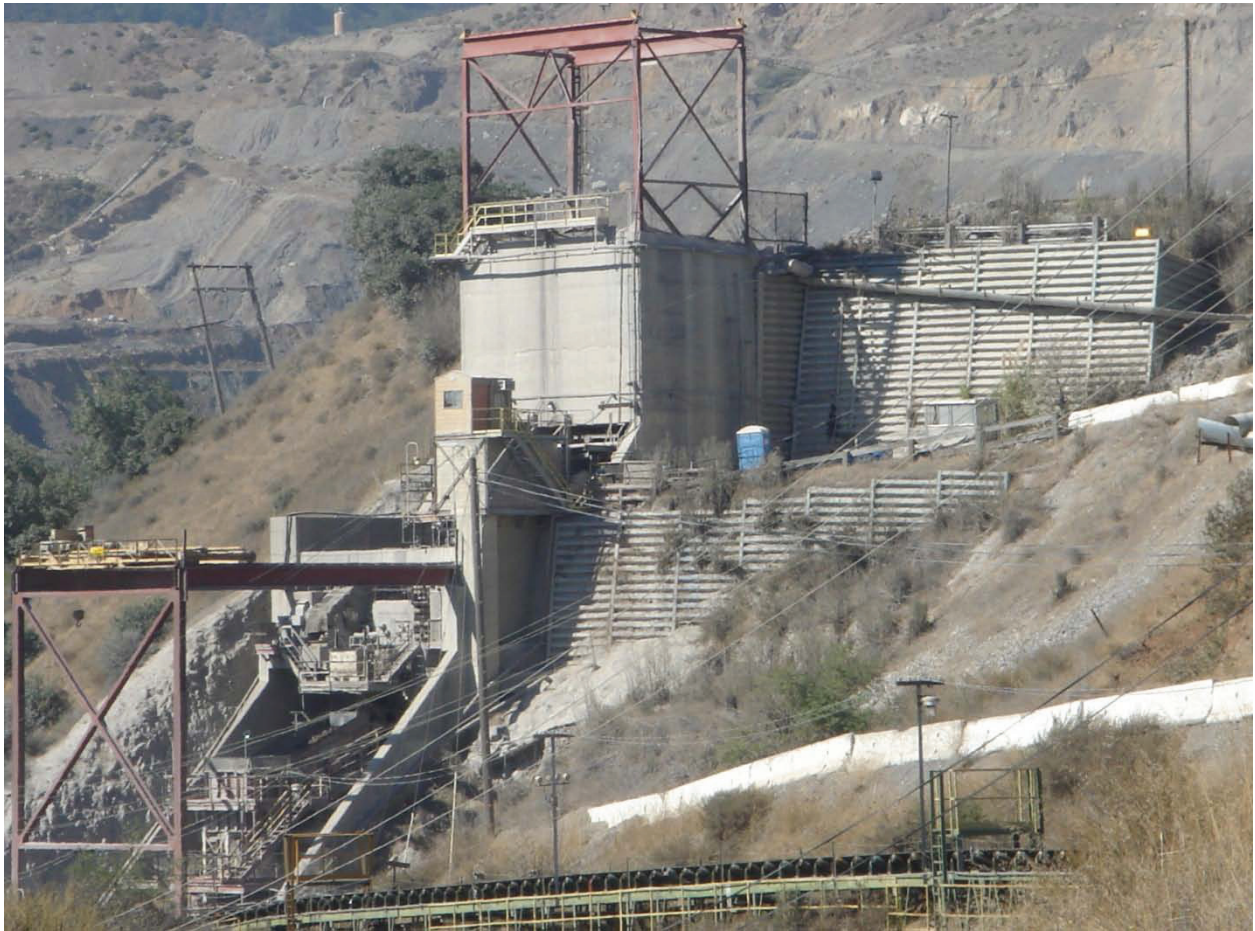
Picture 1 Primary Crusher
