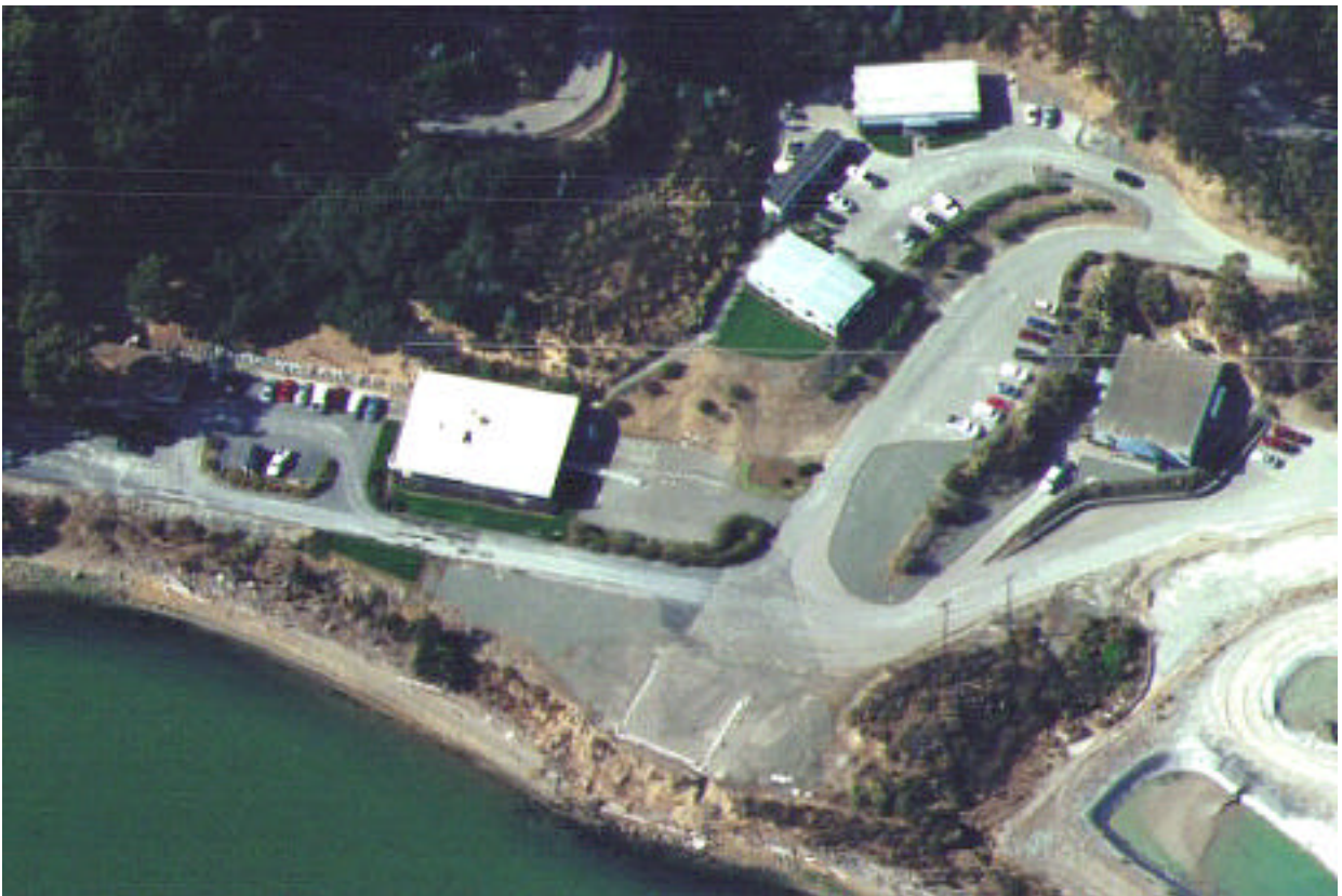
San Rafael Rock Quarry - Office Complex
