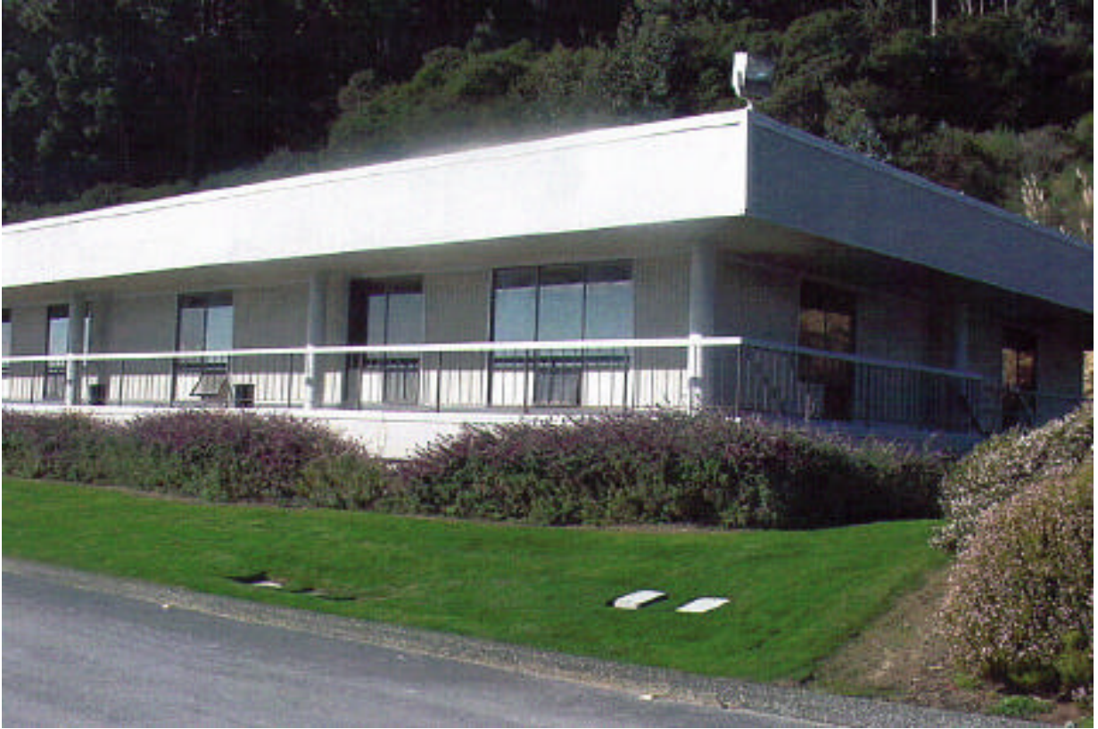
San Rafael Rock Quarry Office Building
